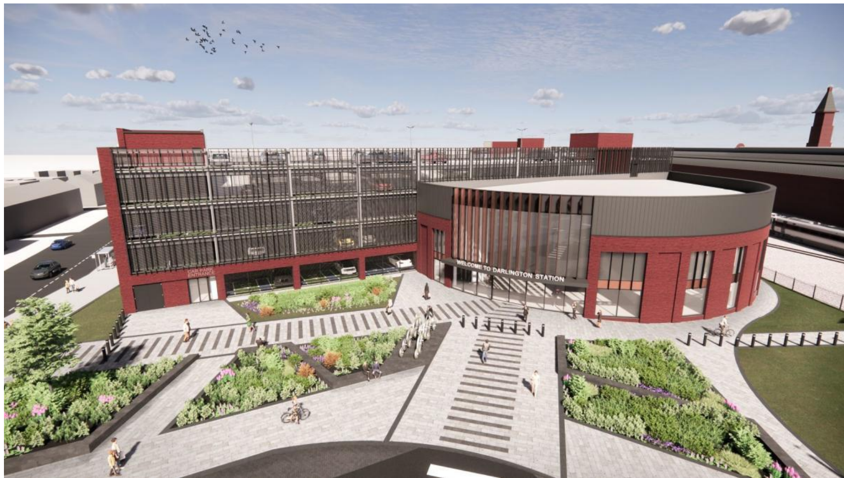
View looking southwest towards the new station entrance
